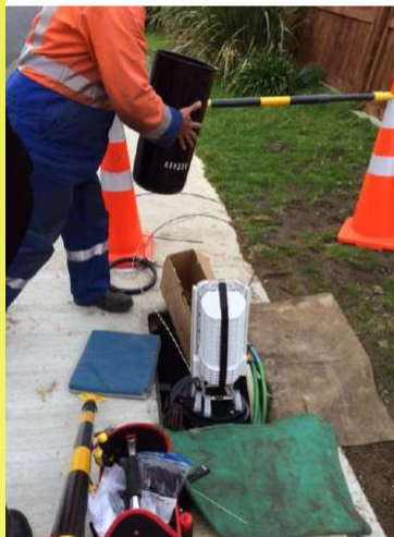
Chorus U/g splitter 16:1 fibre splits x3
