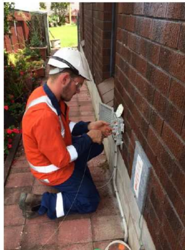
NP Install external termination point
