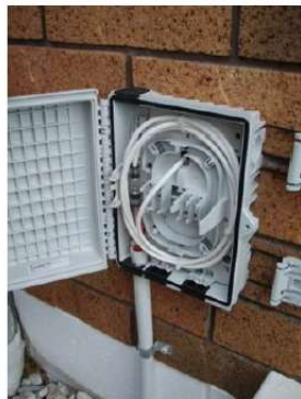
External termination point on house where fibre enters the house
