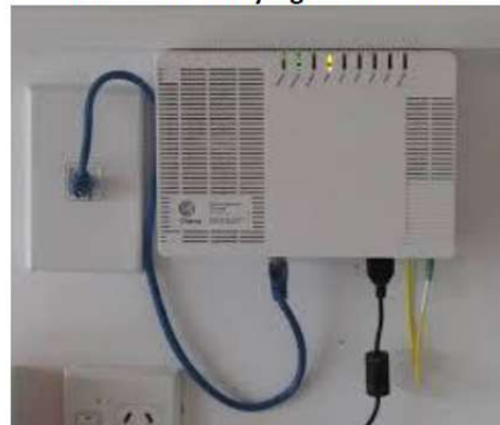
Optical termination unit (ONU) converts optical light to Ethernet in the home
