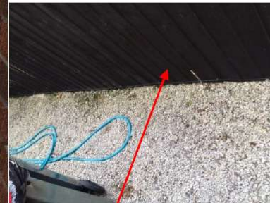
Fence Line Install
