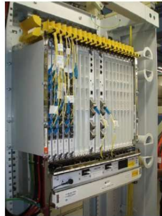
Optical Line Terminal (OLT) Optical equipment that "light" the fibre with lasers to carrying internet data
