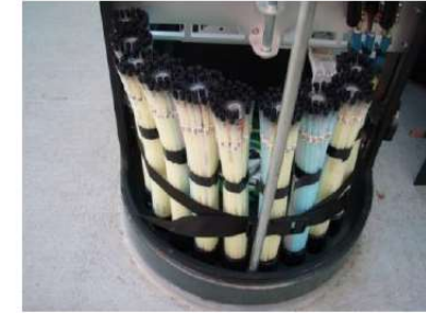
Micro ducts in cabinet Fibre is blown through micro-ducts to the home
