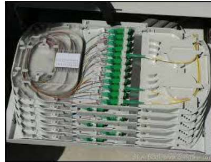
Optical splitter in cabinet Light from a single fibre is split 24:1 to 24 individual fibres for each house
