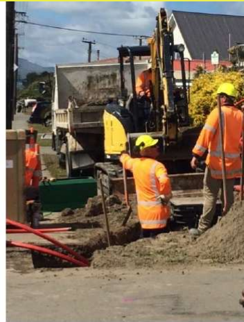
Cabinet installation CHCH
